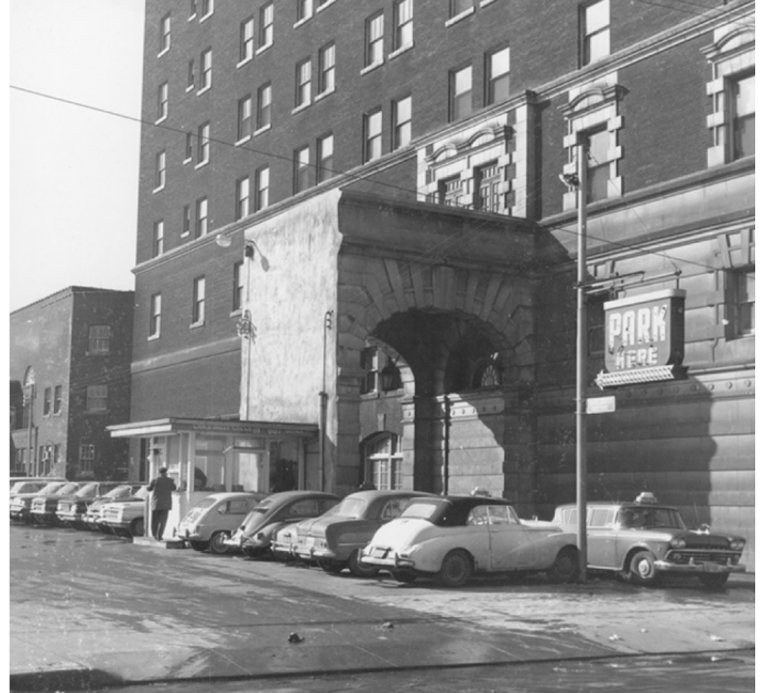
A view of the side of the building at the intersection of King St. and Catherine St. in 1960. The view from here is quite similar today.
