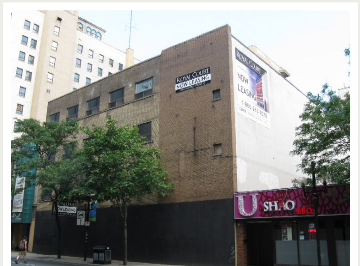
View of the building around 2012 before current construction began.
