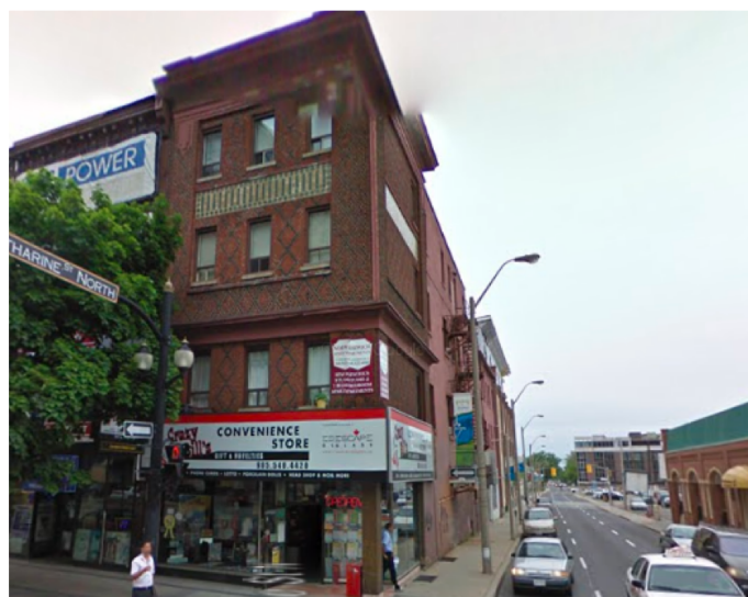
The building as it looked in 2007. It looks very similar to how it did in the 1950s. The building is currently under renovations to become the Gore Park Lofts.
